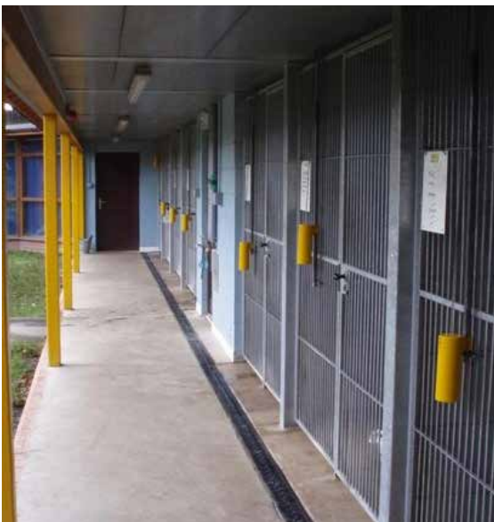
Protected external runs (showing drainage)
